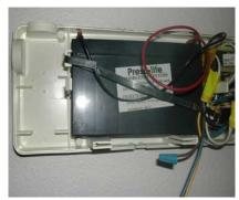
If the Emergency light fails to operate when the test button is pushed, more than likely the battery has failed (but remember to also check the bulbs). All emergency lights have an internal battery and battery charger. Replacement Batteries can be purchased at Grainger's or City Lighting.
